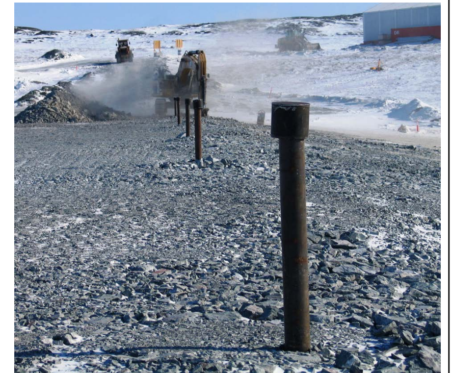
Survey monitoring points installed along upstream crest of dam, April 16, 2012
