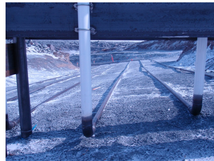
Connection between thermosyphon piles and radiators for South Thermosyphon Radiators, April 17, 2011
