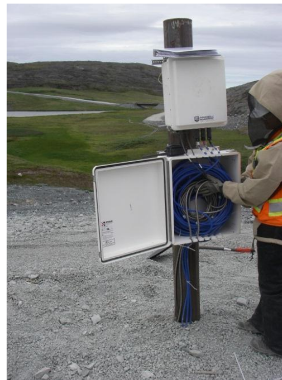
Lead cables were coiled up and placed into the cable management boxes immediately below the instrument housing.
