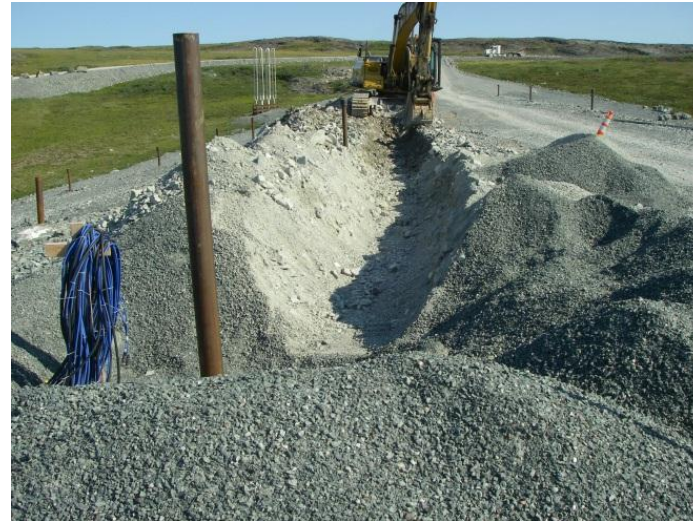
Excavating cable trench between ISP 085 and ISP 130. Photo looking north-east along the dam crest. Note the settlement monument (mid-was avoided when excavating the trench.
