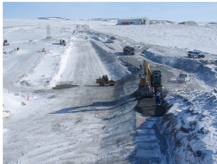
Placement of core material in Fillet Zone (pre liner ), April 23, 2011
