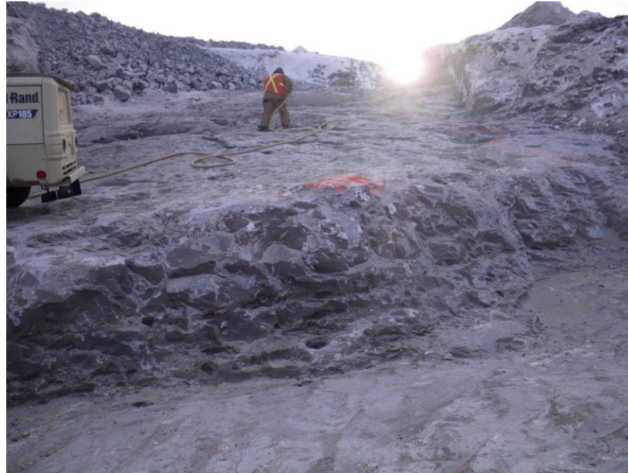
Labourer using air compressor to clean base of Key Trench, March 16, 2011
