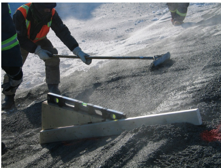
Device for setting slopes, labourers hand sloping the upstream face of the core, February 26, 2012
