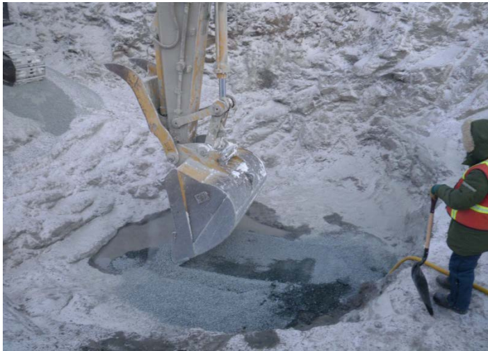
Failed first attempt at mixing-in-place core placement in Peat Zone excavation, February 24, 2011
