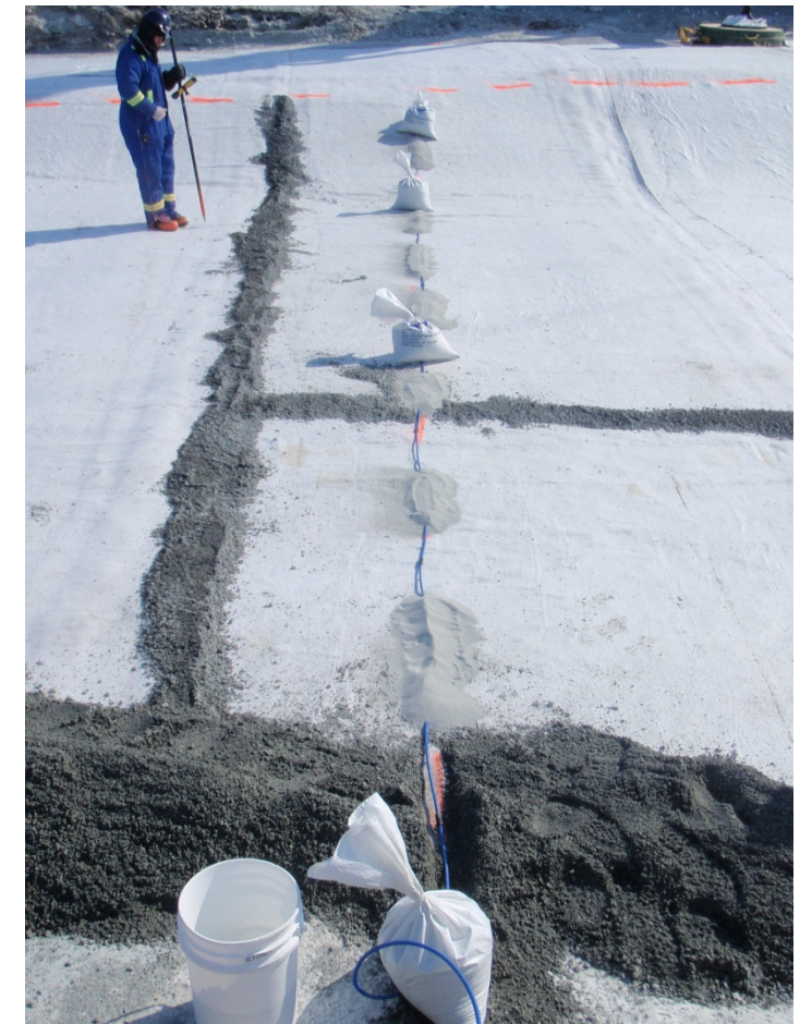
Placement of horizontal GTC on surface of lower GCL, April 25, 2011
