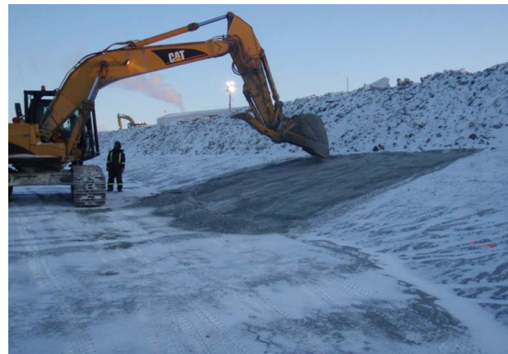
Removal of thermal cover: excavator scraping frozen 16 mm clear material from frozen core material surface, January 25, 2012
