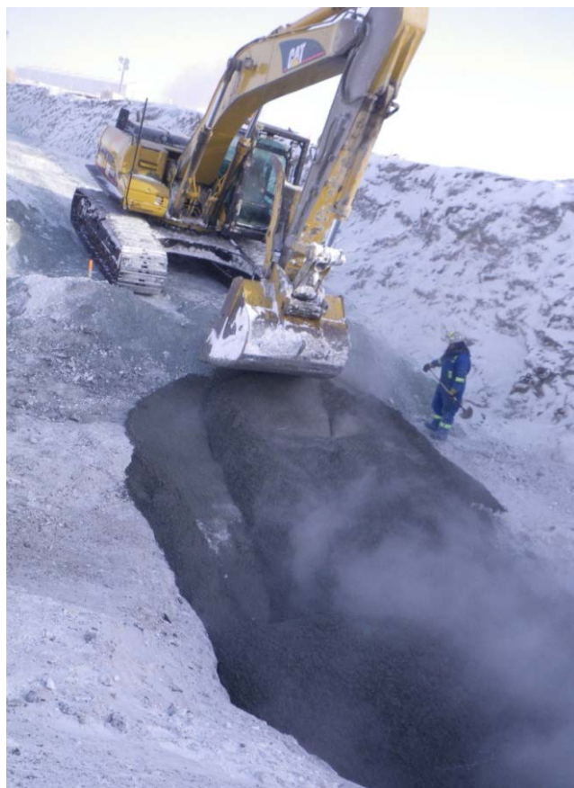
Placement of core material on the edge of the Peat Zone over-excavation, March 9, 2011
