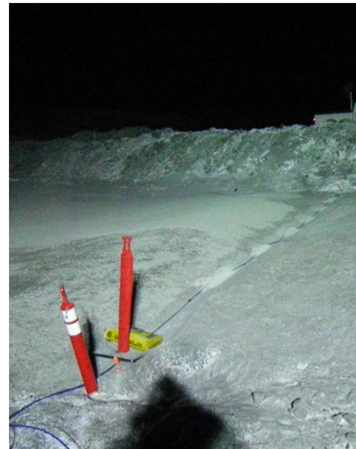
Installation of horizontal GTC in small trench, February 9, 2012
