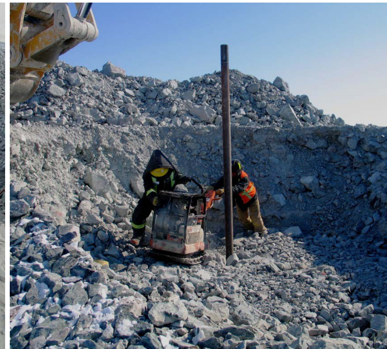
Compaction of first lift of material around crest survey monument pipe, April 17, 2012
