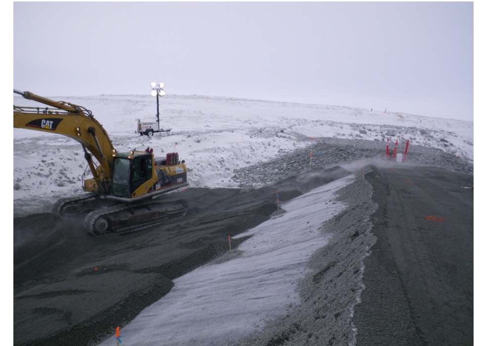
Placement of GCL cover material on the upstream slope of the core, March 31, 2012
