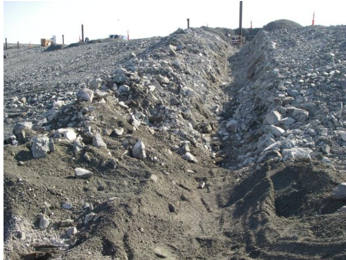
Cable trench excavated for thermosyphon status thermistors lead cables. Photo taken from south Thermosyphons looking east toward ISP 040.
