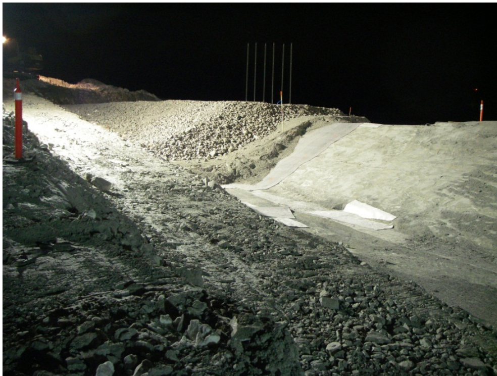
Staged construction; lift of transition material over GCL cover material, March 29, 2012
