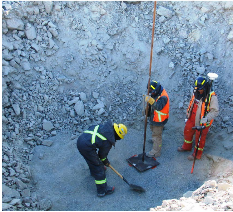
Installation of the inner rod of crest survey monument point on downstream side, April 18, 2012
