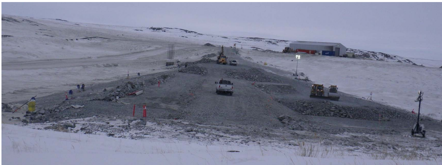
Staged ROQ construction, photo looking northeast along dam alignment, April 2, 2012
