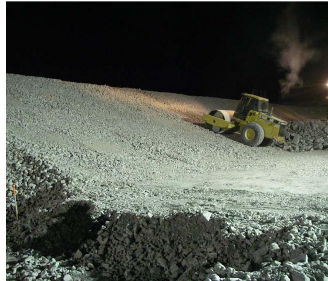
Compacting transition material along upstream slope of core, March 27, 2012
