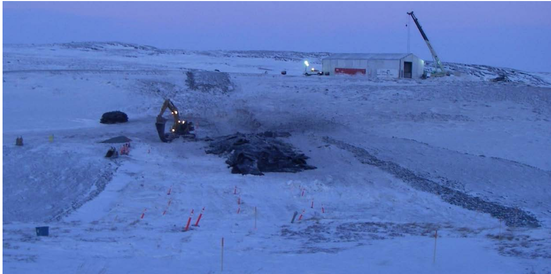
Removal of blast mats after Key Trench blast, photo looking northeast, February 5, 2011
