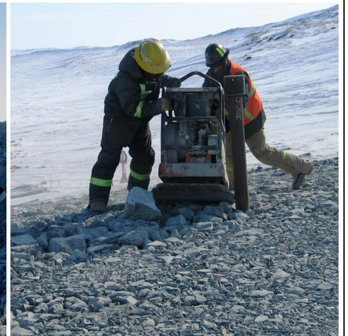
Compaction of last lift around crest survey monument pipe, April 16, 2012
