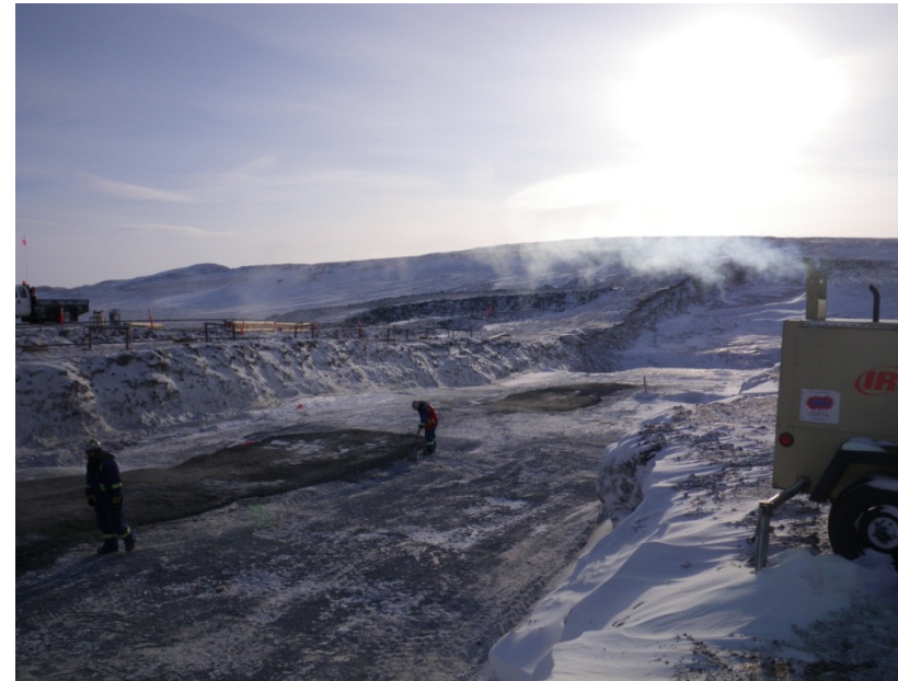
'Test pads' of blended core material placed within the dam footprint, bleeding of water still occurring. Photo taken March 6, 2011
