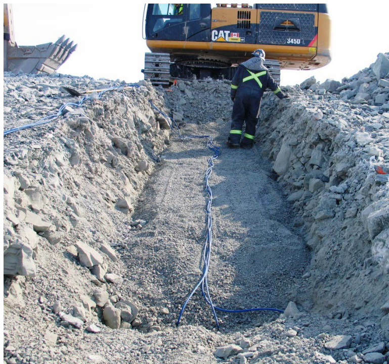
Bedding of cable cluster at station 0+40 along the downstream side of the dam, April 19, 2012
