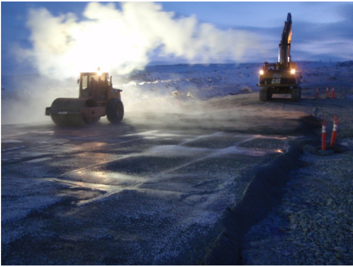
Compaction of core material, February 22, 2012
