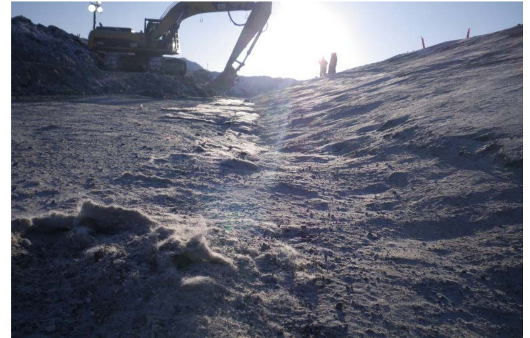
Damage to lower GCL due to the removal of thermal cover material, March 23, 2012
