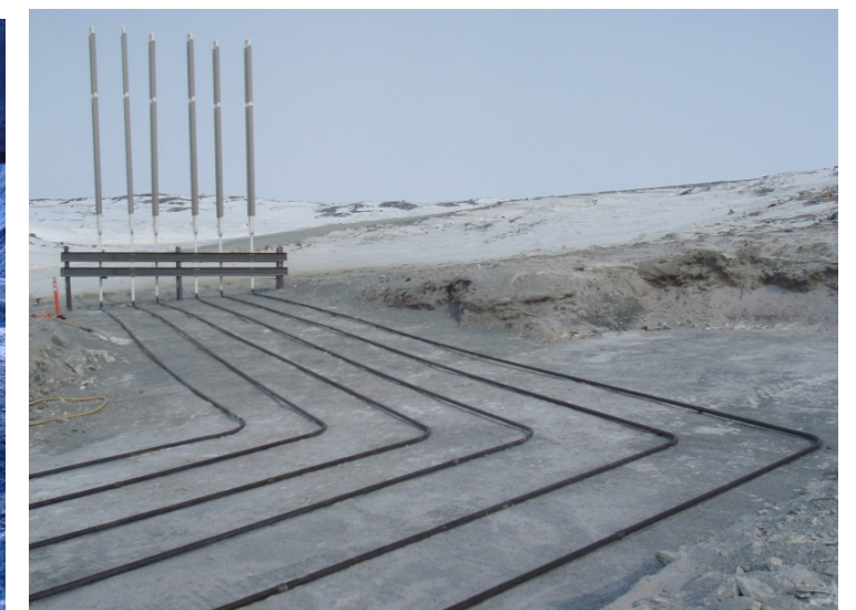
Thermosyphon pipes running to North Thermosyphon Radiators, April 19, 2011
