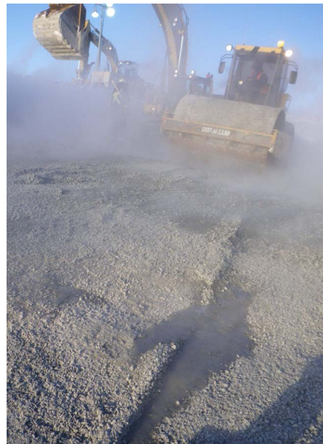
Excessive bleed water was noted during levelling course placement with the original (20 mm minus) core material. Photo taken March 3, 2011
