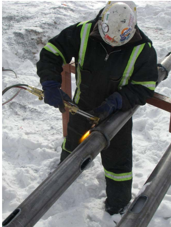
Welding piles for thermosyphon radiators, April 2, 2011
