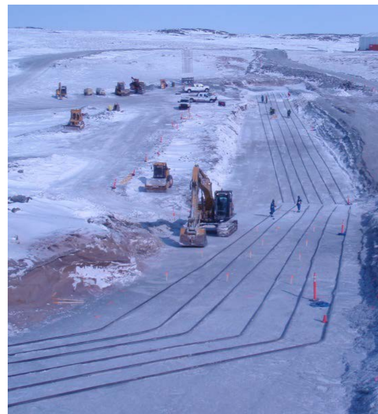
Thermosyphon pipes laid out in Key Trench, photo looking northeast. Photo taken April 17, 2011
