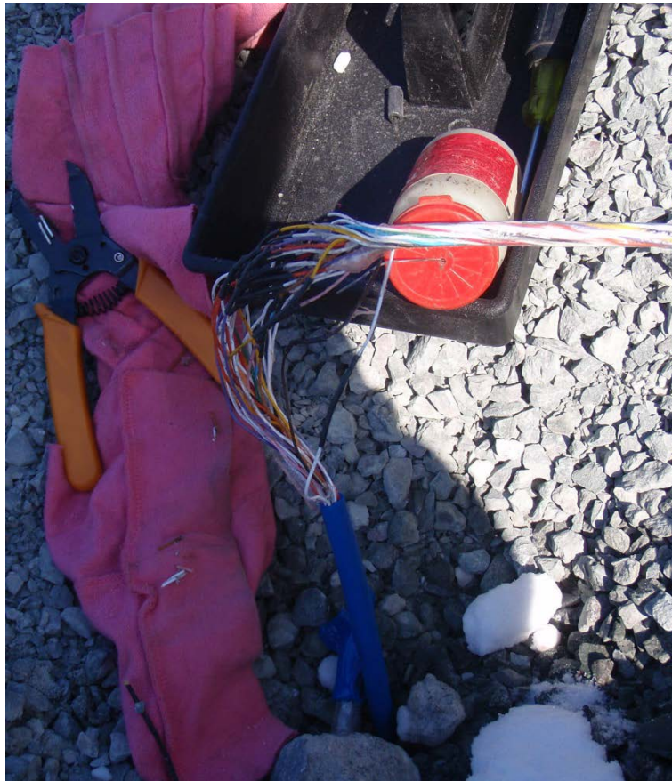
Splicing damaged GTC, April 29, 2011
