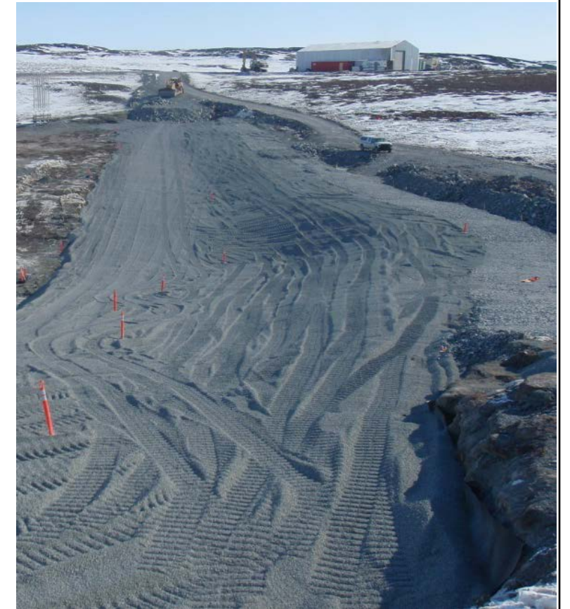
Thermal cover placement: placement of 16 mm clear indicator material complete; placement of ROQ started, May 6, 2011
