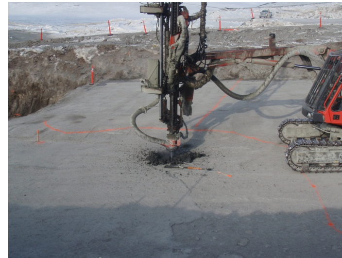
Drilling for installation of vertical Key Trench GTC, April 29, 2011
