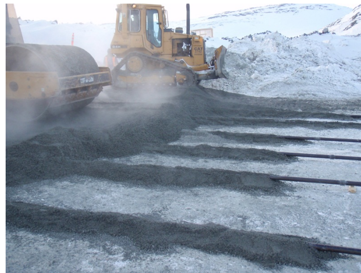
Covering thermosyphon pipes with core material, April 17, 2011
