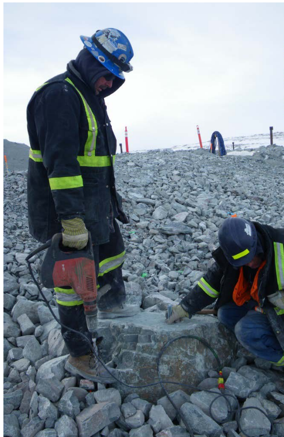
Installation of pin for surficial survey point, May 6, 2012
