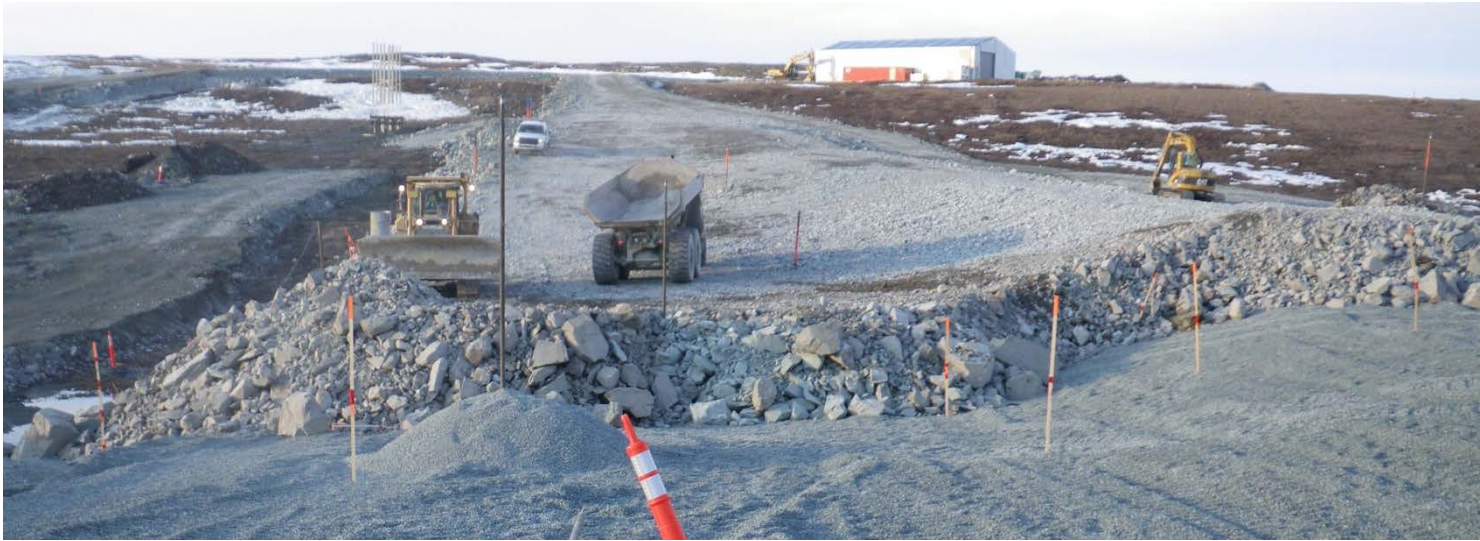
Thermal cover placement: placement of ROQ material for thermal cover, thermistor strings protected with steel pipes, May 14, 2011
