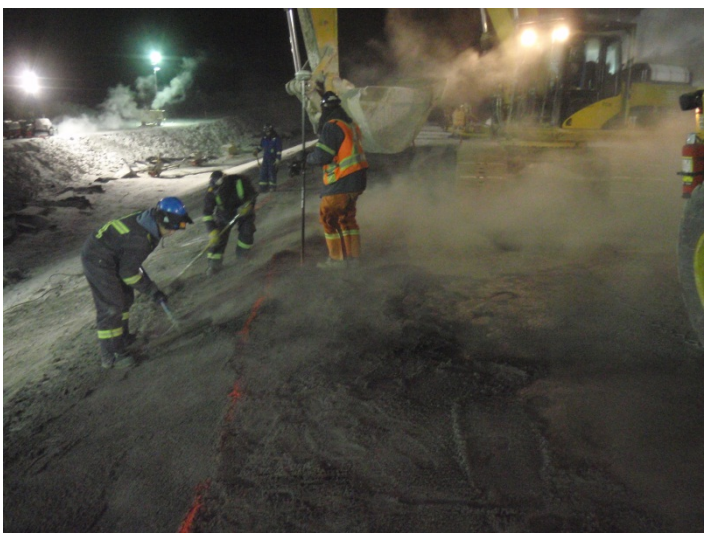
Labourers sloping the upstream side of the core, March 10, 2012
