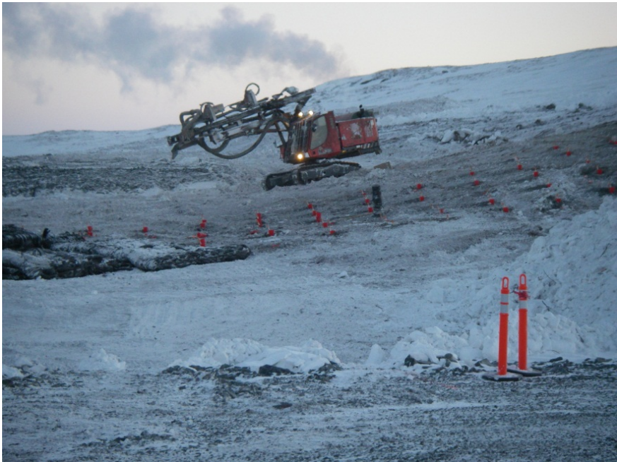
Drill on blasting pattern for dam, February 9, 2011
