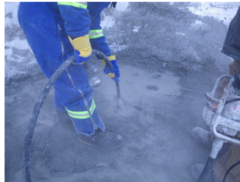
Compaction of core material with a concrete vibrator in an area which could not be accessed by the roller compactor. Photo taken March 11, 2011
