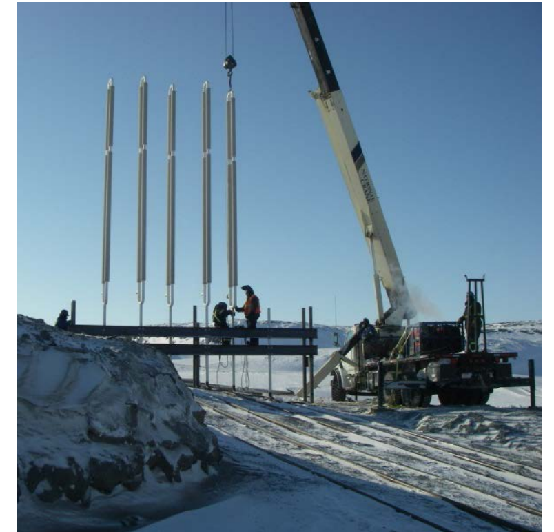
Installation of South Thermosyphon Radiators, April 9, 2011
