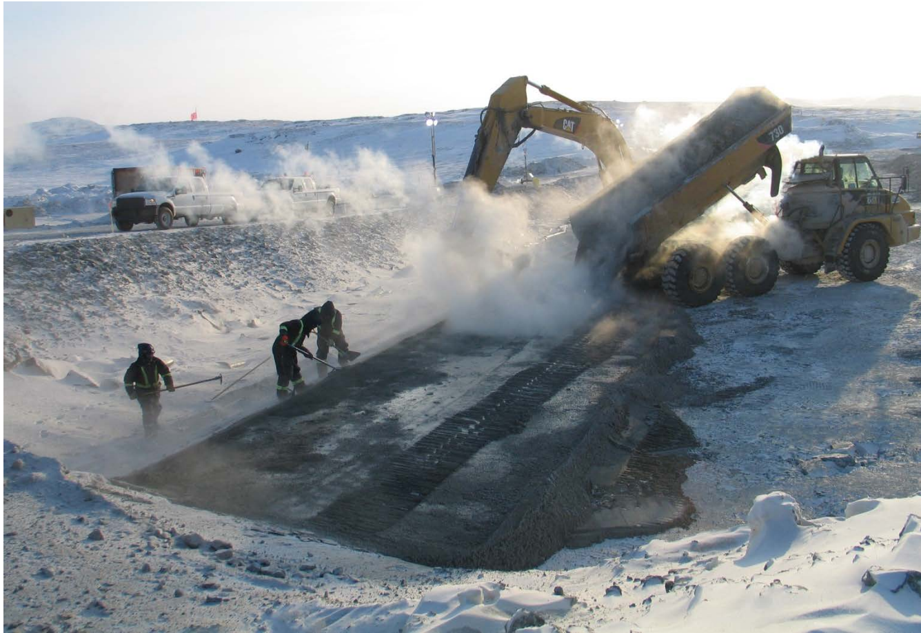
Placement of core material, photo facing south, March 8, 2012
