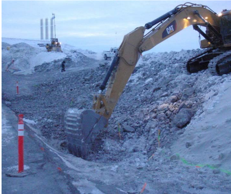
Placement of transition material to form access ramp on downstream side of core, February 1, 2012
