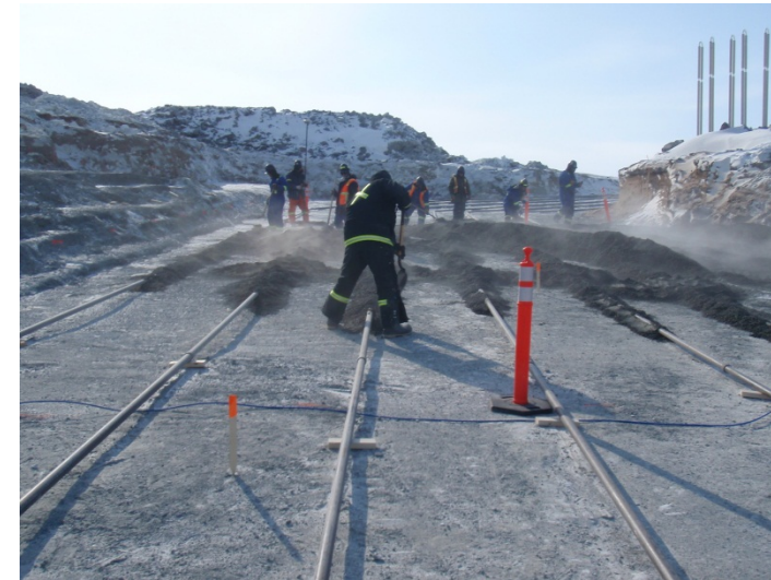
Labourers spreading core material over the thermosyphon pipes prior to core material placement with bulldozer, April 17, 2011
