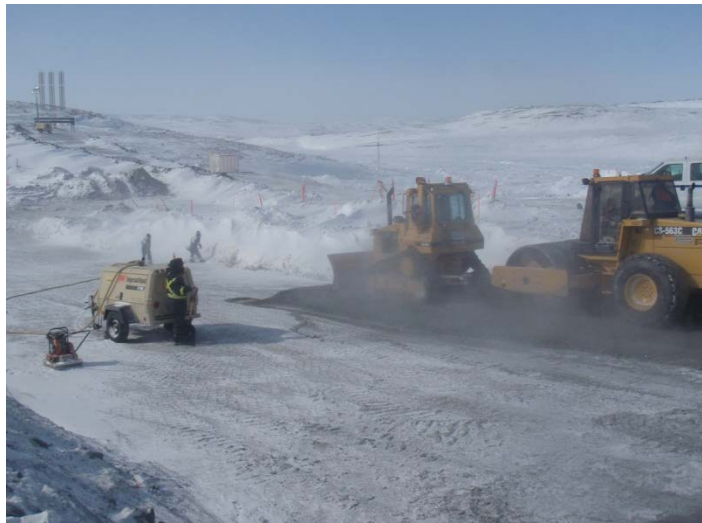
Core material placement with CAT D4 bulldozer, April 21, 2011
