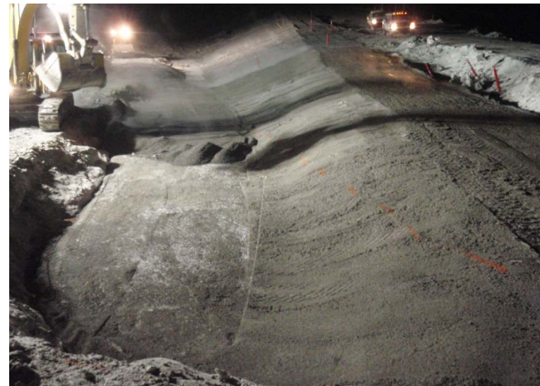
Placement of GCL cover material along toe of upstream slope, March 20, 2012
