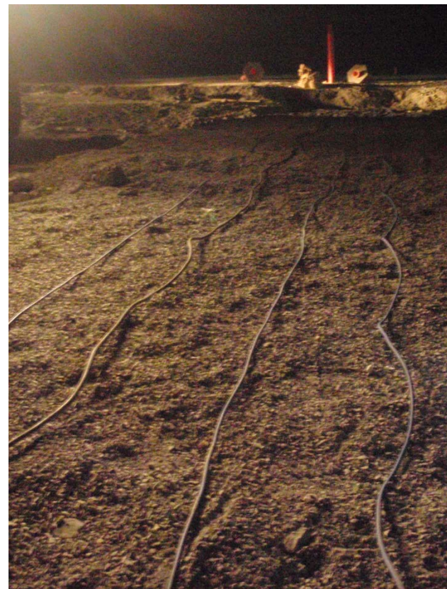
Laying out GTC cluster towards the downstream at station 0+85, preparation for covering, March 15, 2012
