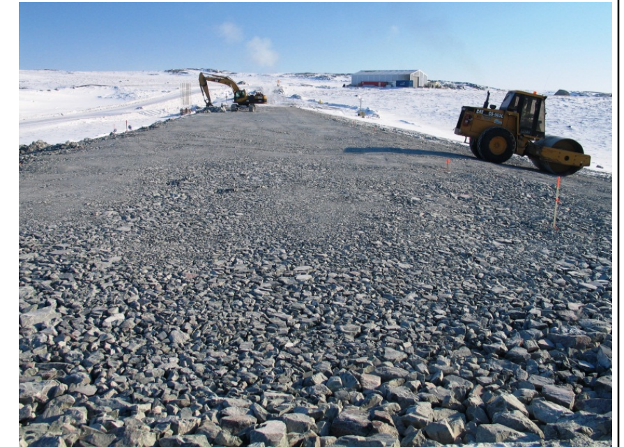
Excavator sloping ROQ on downstream side and packer running on upstream side, April 8, 2012
