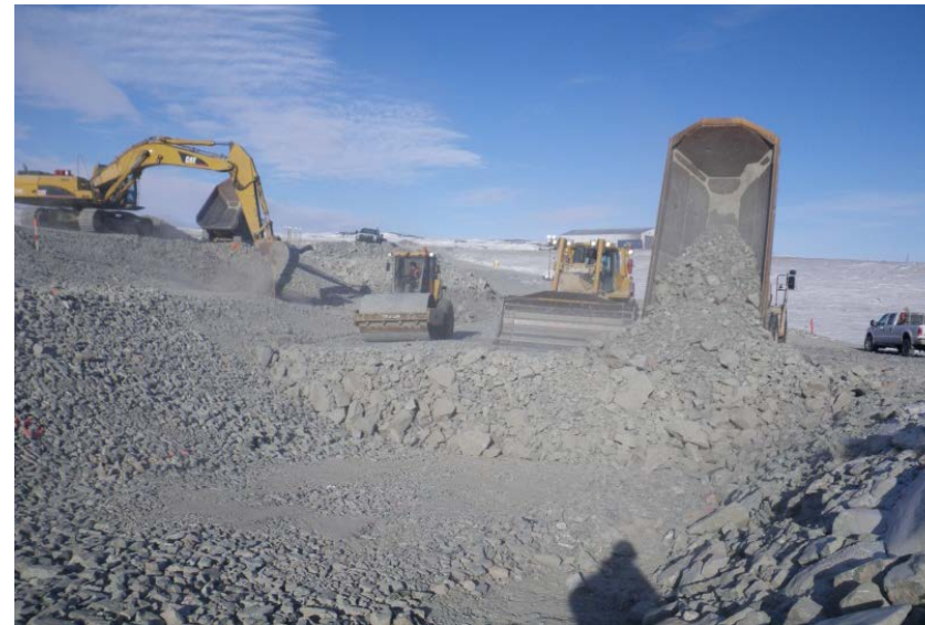
Staged ROQ placement along upstream side of dam, April 1, 2012
