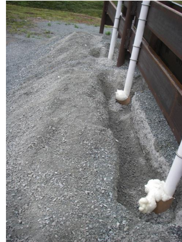
Thermosyphon status thermistors were heat-insulated using expanding spray foam.
