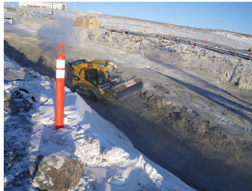
Cleaning of Key Trench after removal of non-spec. core material, March 12, 2011
