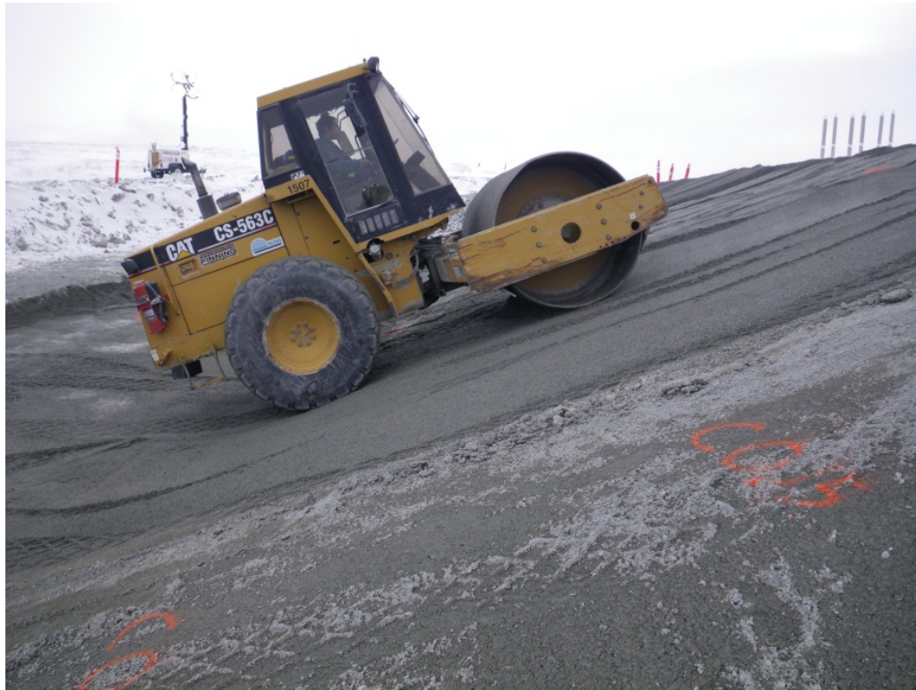
Compaction of GCL cover material, March 31, 2012. Note the survey grade marks in the foreground
