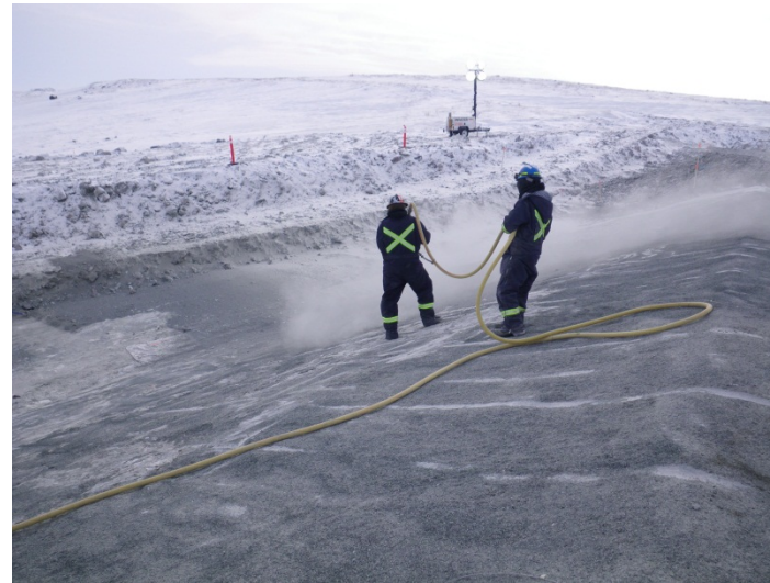
Cleaning debris off upstream slope of frozen core prior to GCL placement, March 30, 2012
