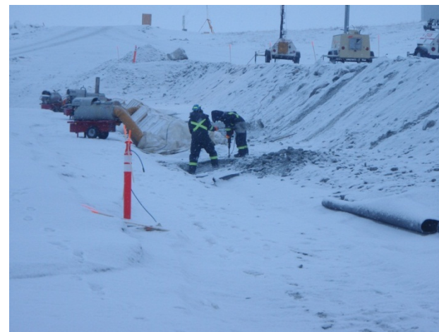
Thermal cover removal: labourers using a small jackhammer to remove frozen 16 mm clear material from above the lower GCL
