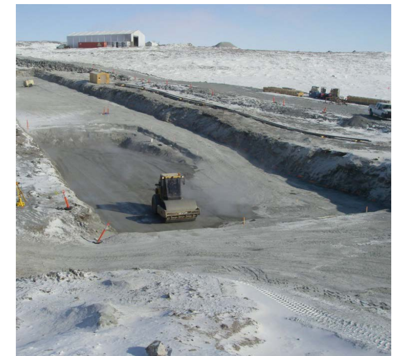
Vibratory compactor compacting core material placed in the low area created by the excavation of hyper-saline material in the Soft Spot, April 3, 2011
