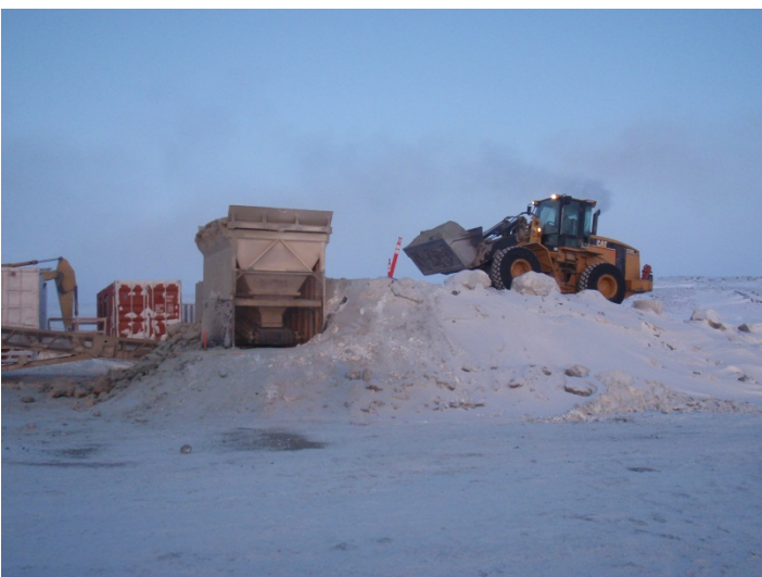
Loader loading dry core material into Frozen Core Plant hopper, January 21, 2012
