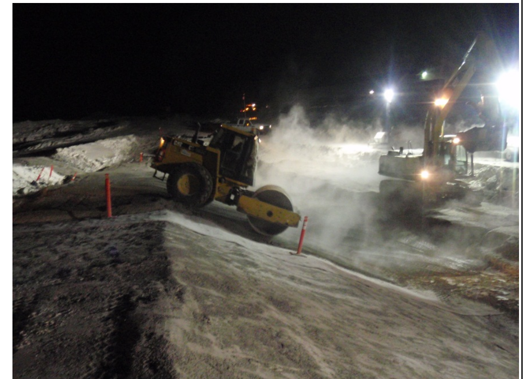
Compaction of GCL cover material along the slope of the core, March 20, 2012
