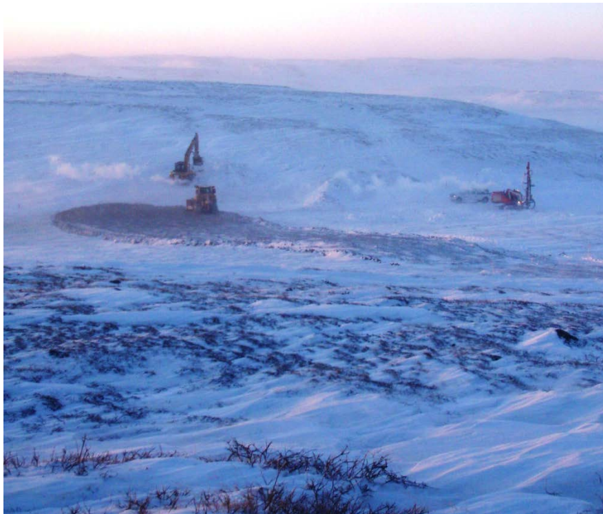
Placing first lift of ROQ, January 25, 2011
