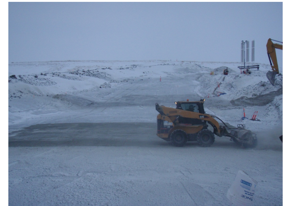
Cleaning snow and debris from surface of frozen core prior to placement of next lift, January 31, 2012
