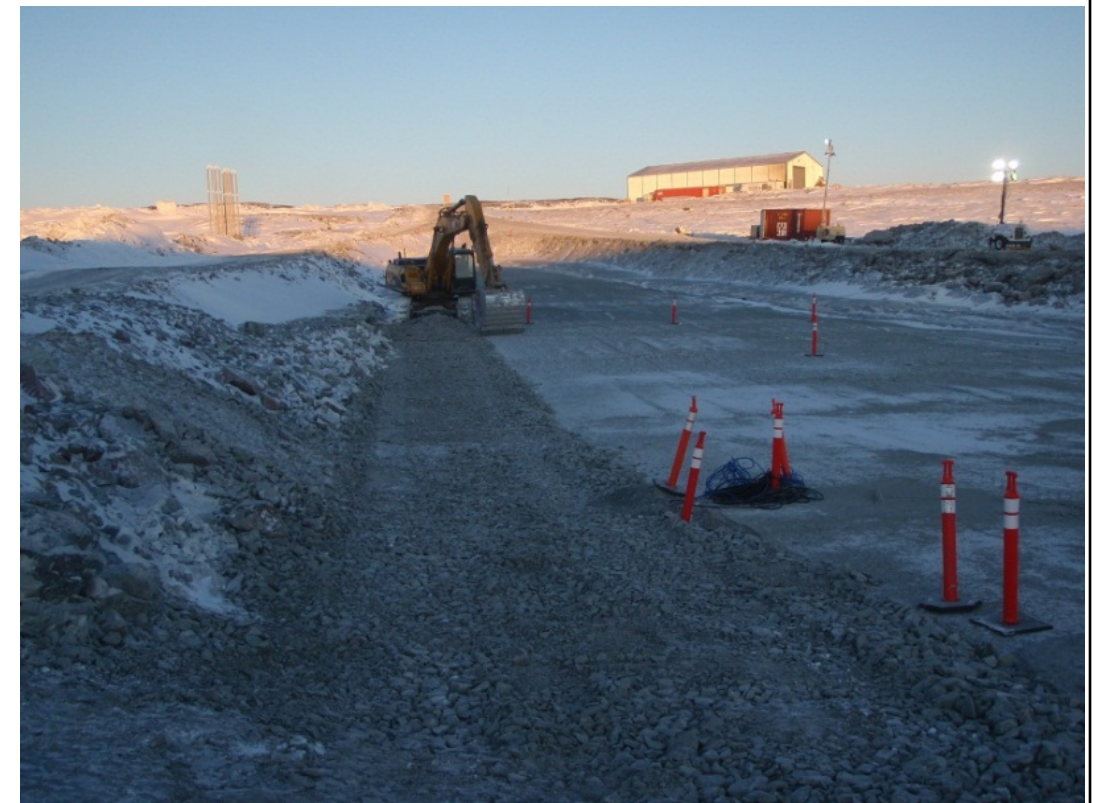
Placement of transition material on downstream side of core, February 9, 2012
