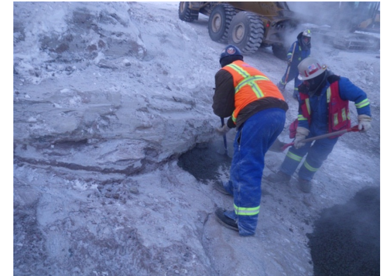
Labourers shoveling core material into holes at the base of the Key Trench, March 7, 2011
