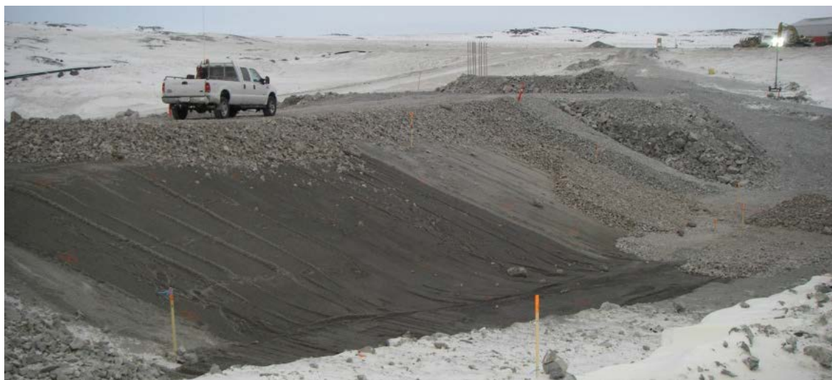
GCL cover material placement completed, March 31, 2012
