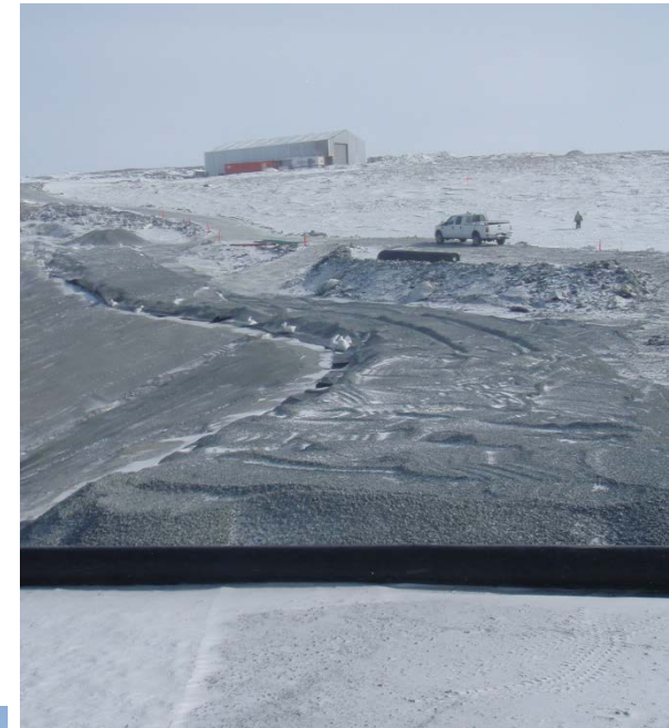
Thermal cover placement: HDPE liner covered with 16 mm clear material overlying exposed lower GCL, April 30, 2011
