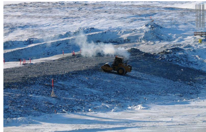
Compactor packing downstream slope of dam, March 12, 2012
