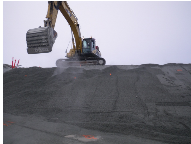
Placement of GCL cover material with CAT 330 excavator, March 31, 2012
