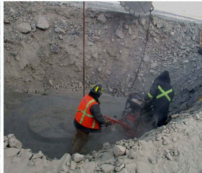
Compaction of crush material over steel plate of crest survey monument, April 15, 2012
