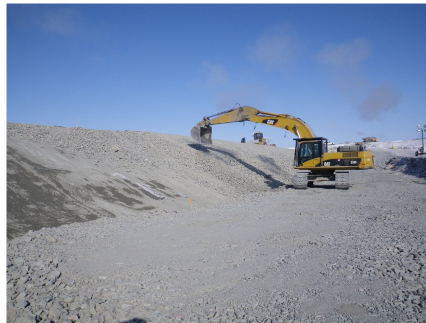
CAT 345 excavator placing lift of transition material along upstream slope of core, March 26, 2012
