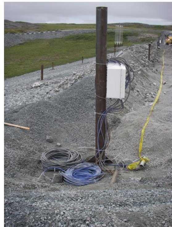
Excess cable was coiled up and buried at the base of the instrument support post. Photo taken from ISP 085 looking north-east along the crest of the dam.
