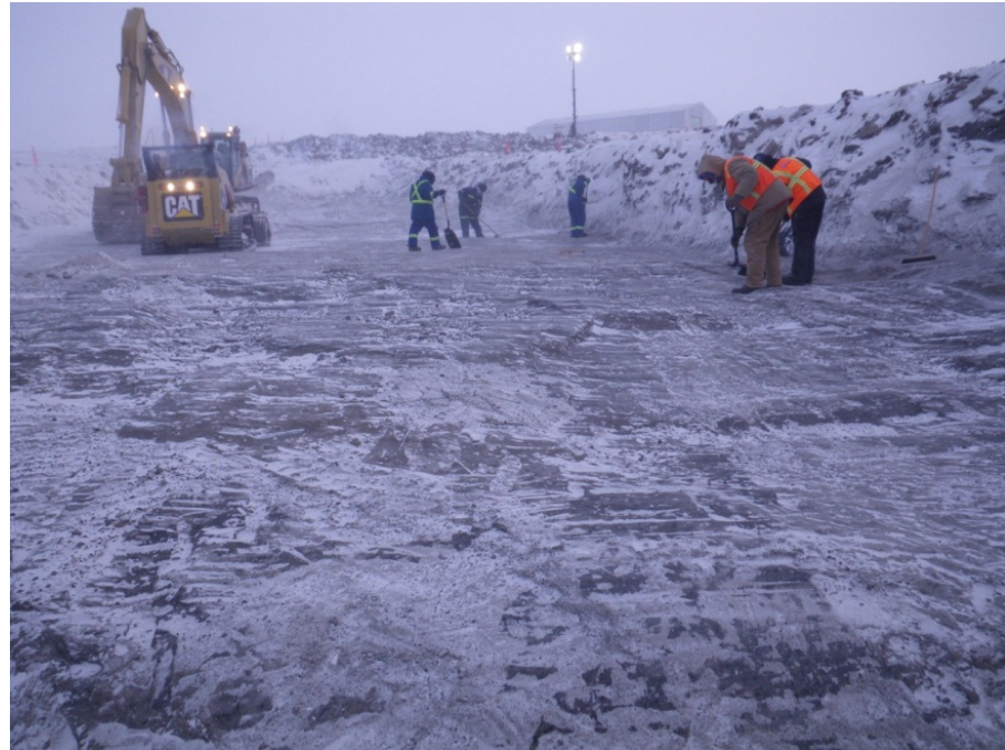
Labourers, excavator, and skid steer with broom attachment cleaning base of Key Trench north of inflection point, February 28, 2011
