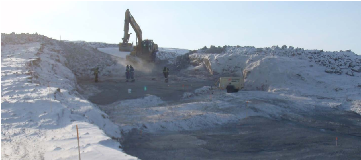
Placement of levelling course on south end of dam, March 18, 2011
