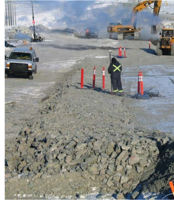
Placement of transition material along downstream side of core, March 3, 2012
