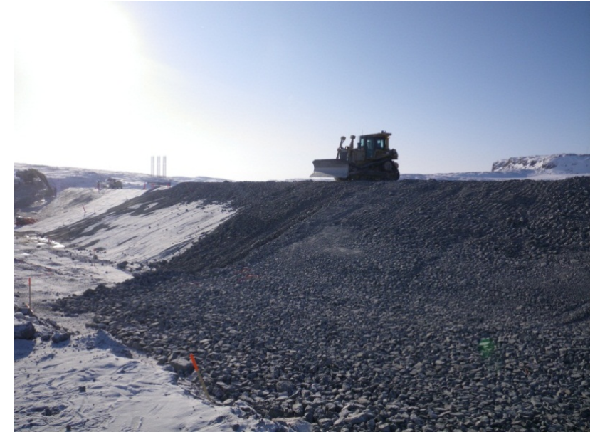
Placement of transition material along the crest of the dam, March 25, 2012
