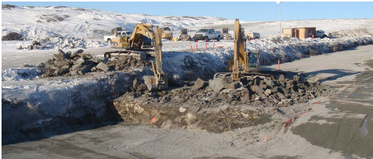
Excavating hyper-saline overburden in Soft Spot, March 22, 2011
