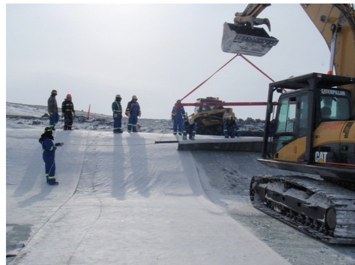
Placement of lower GCL, April 27, 2011
