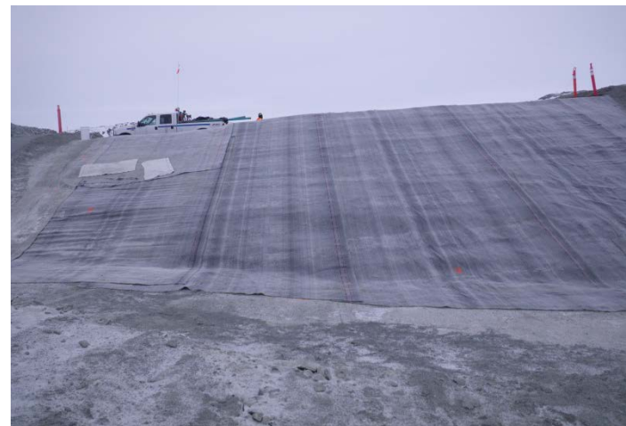
GCL on the upstream slope of the core, March 31, 2012
