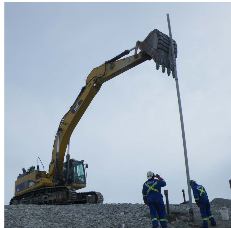
Installation of deep settlement point pipe, May 5, 2012
